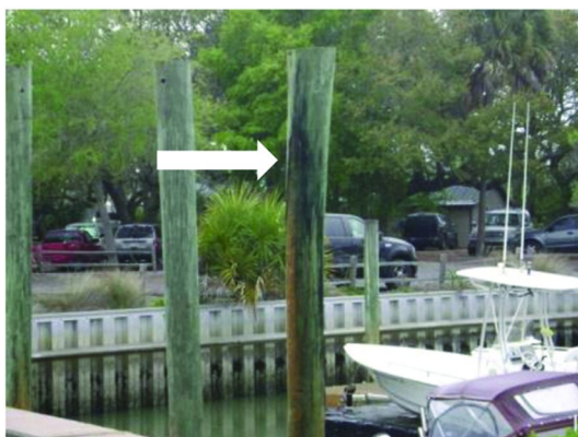
Figure 11. Aureobasidium pullulans growing on a CCA-treated pine piling in a marina in South Carolina. (Courtesy of Jim Healey, Cox Industries by permission.)
