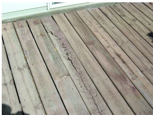
Figure 6. Examples of how once-finished and then unprotected treated-wood decking can experience varying degrees of surface checking and uneven gapping after a 18-year exposure in Wisconsin. (Courtesy of J. Winandy with permission.)
